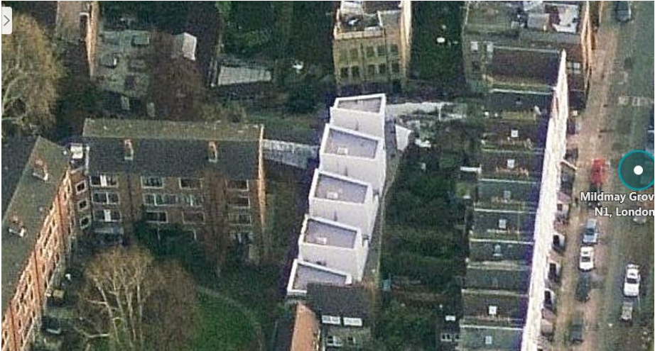
Looking into the site eastwards.
